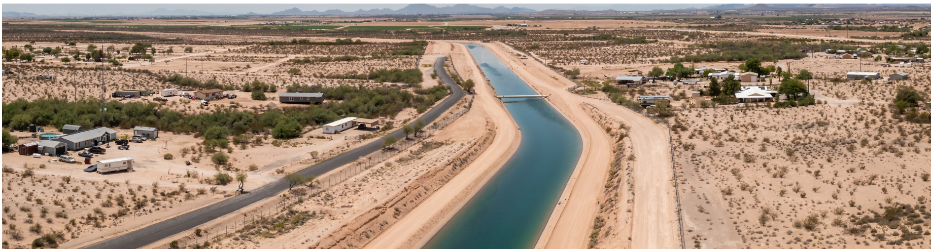
Central Arizona Canal
