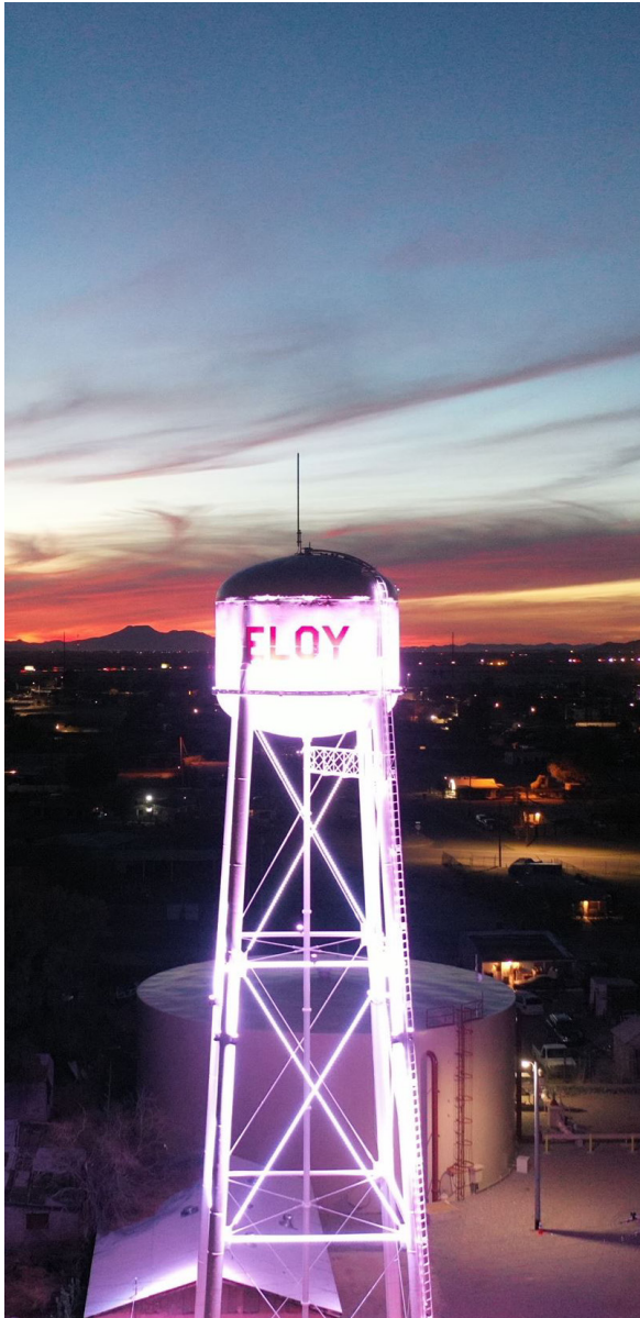
Eloy Water Tower
