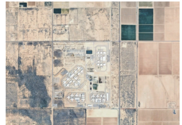
State Route 87 Corridor Growth Area
