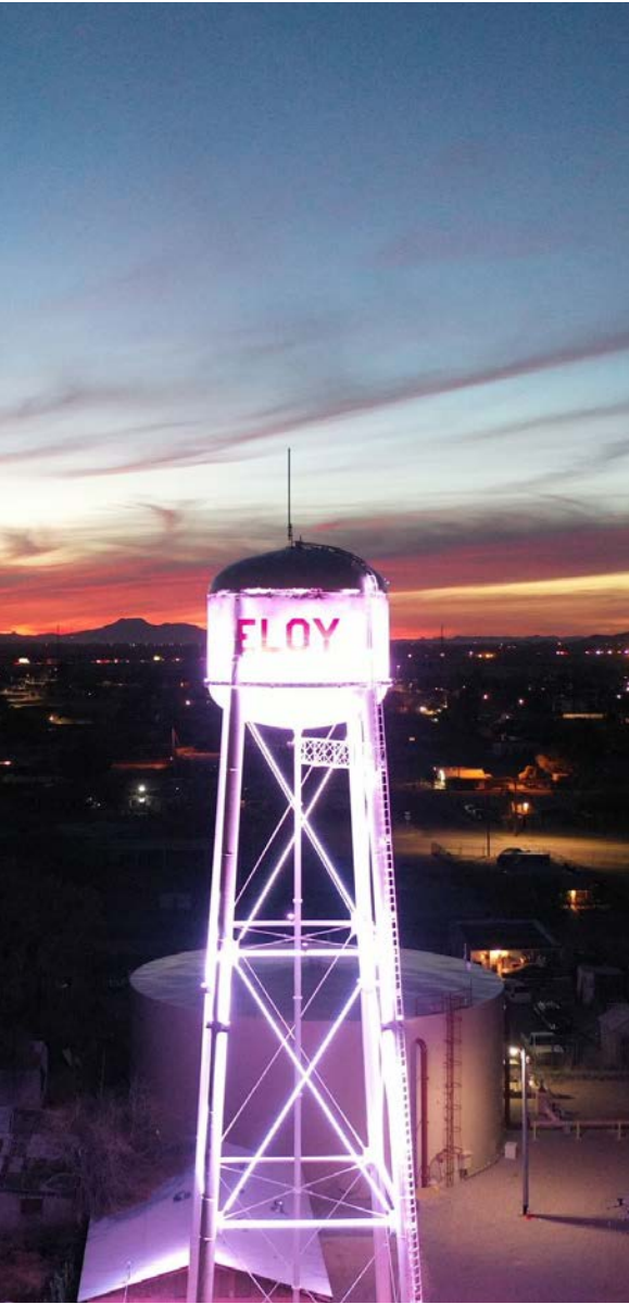
Eloy Water Tower
