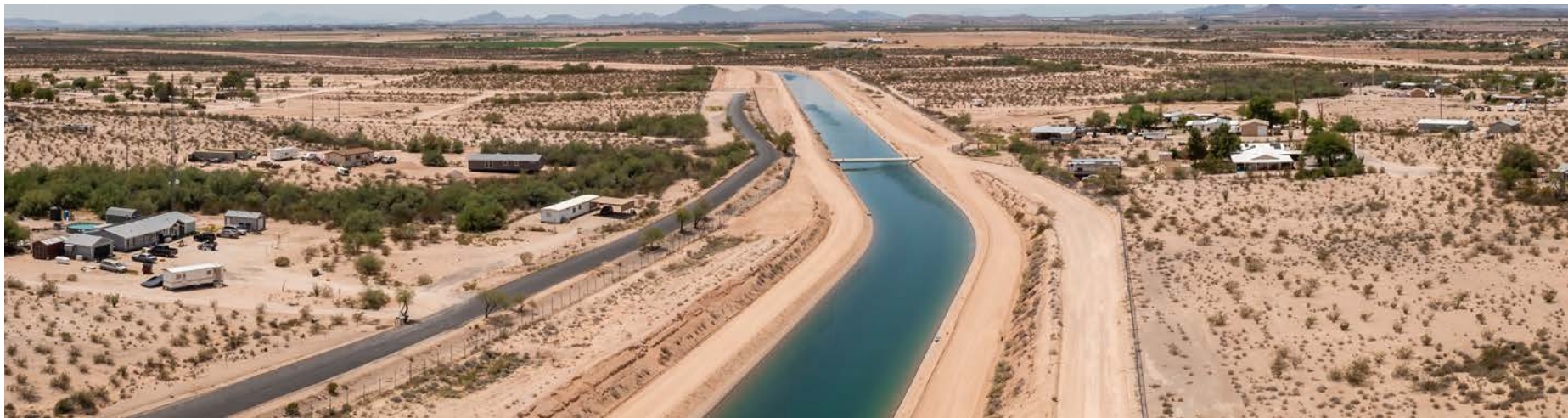
Central Arizona Canal
