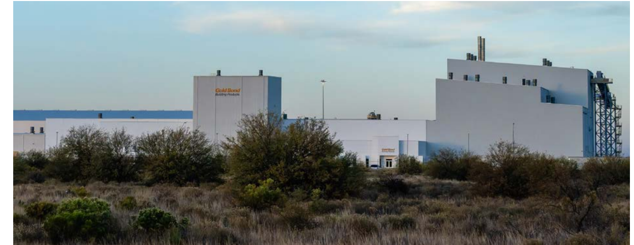
Gold Bond National Gypsum Manufacturing Facility
