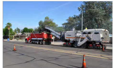
MILLING/PULVERIZING
