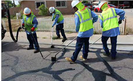
CRACK SEALING
