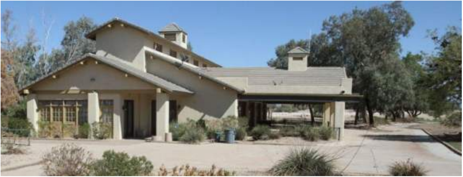
Current abandoned Clubhouse condition
