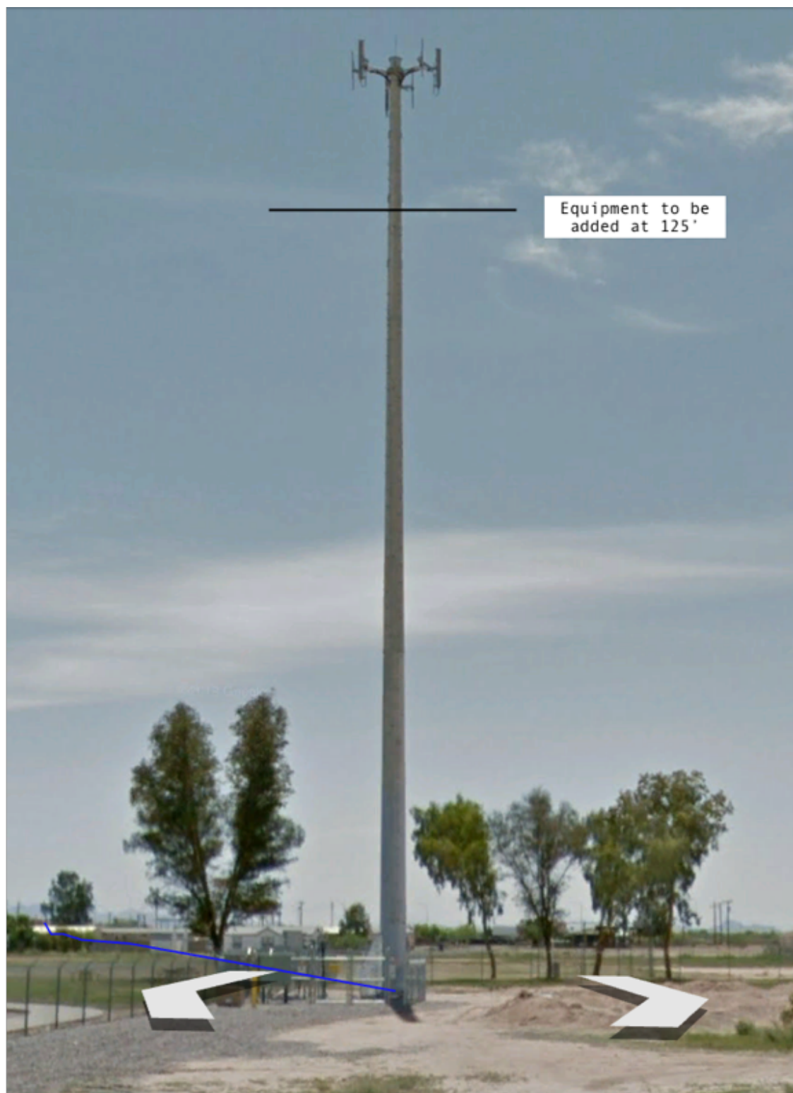
Ground Level Photo of the Monopole in Proposed Condition
